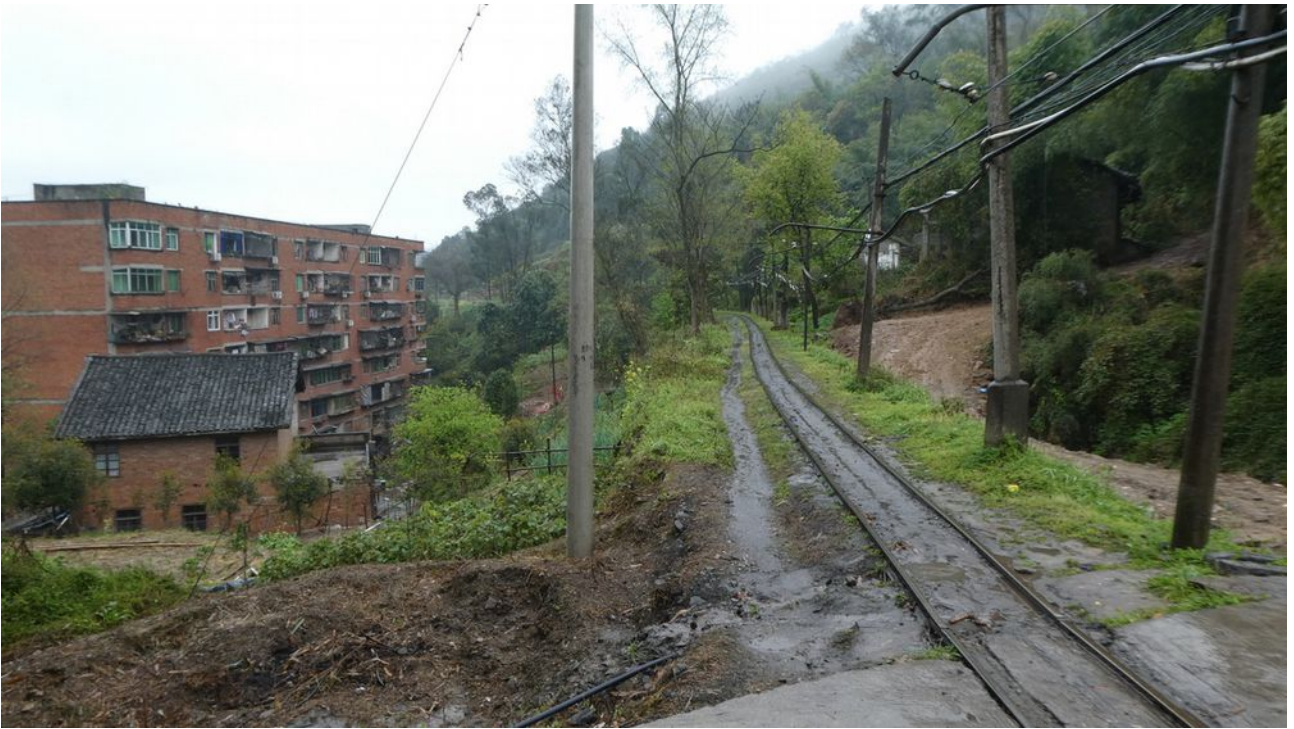
Looking back towards the mine
