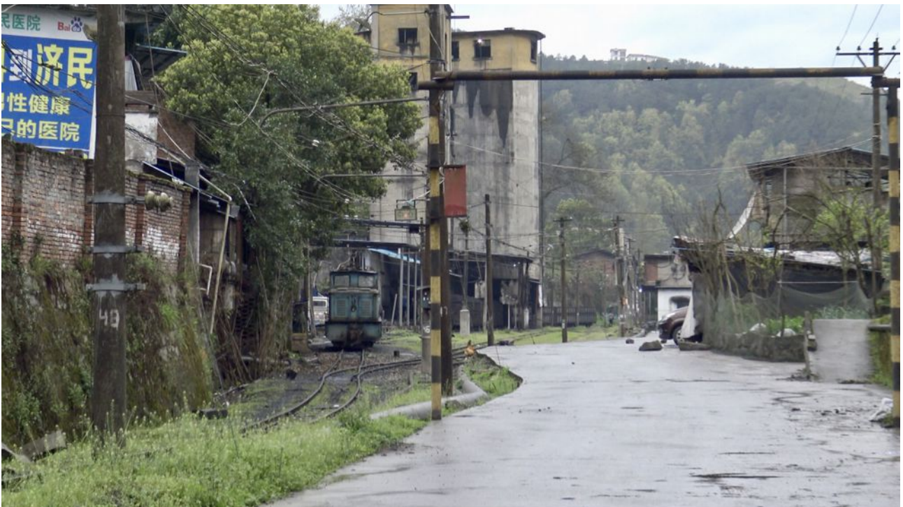
No. 5 waits while its train is loaded by cable at the hoppers.
