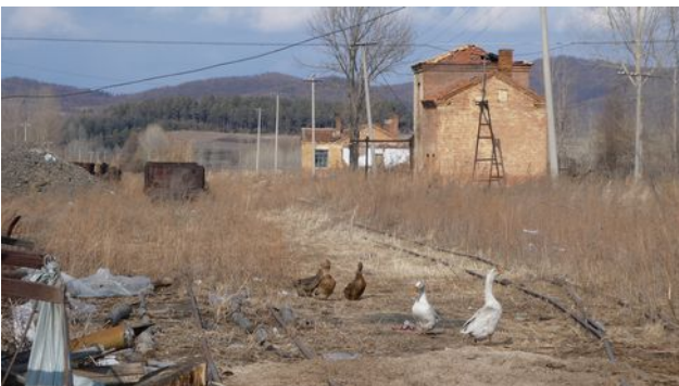
Watering point with the station behind
