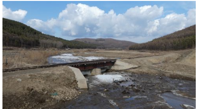
Bridge over stream towards Lishin
